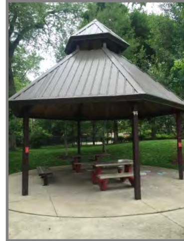
Overall, Park District sitting areas were in “Good” condition. (Field Park)
