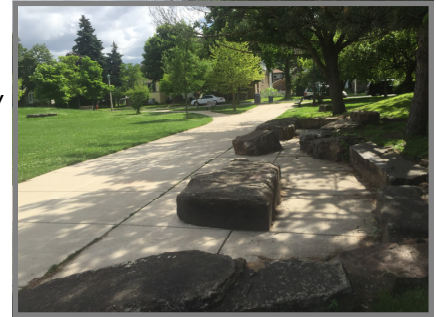
Overall, Park District walkways were in “Good” condition. (Euclid Square Park)
