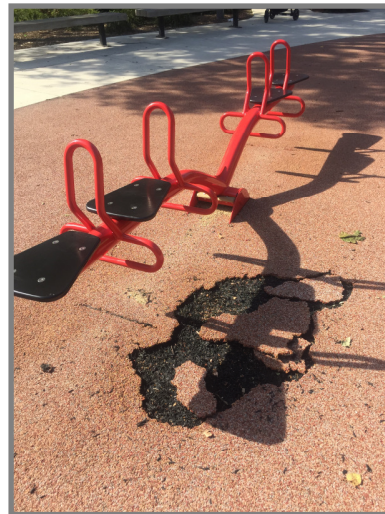
Poured in place surfaces at several playgrounds are starting to show wear. (Scoville Park)
