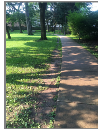
Damage from the snow removal process continues to be an issue with paths & sidewalks. (Lindberg Park)
