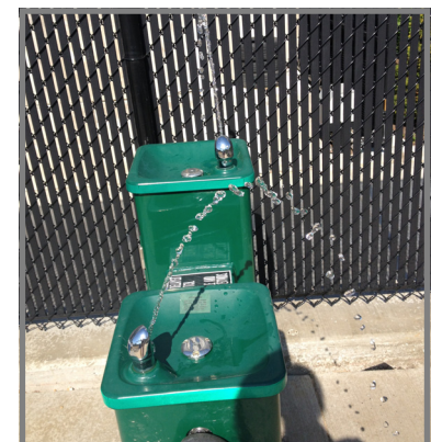
Drinking fountain pressure was either too high or too low in 18% of the fountains evaluated.
