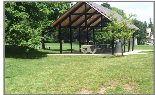
Overall, Park District sitting areas were in “Good” condition. (Taylor Park)
