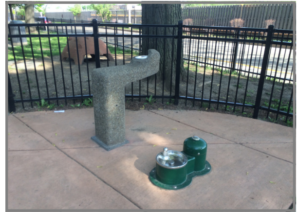
Overall, Park District drinking fountains were in “Good” condition. (Wehnonah Park)
